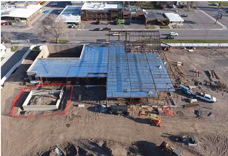
Construction on the Exploration Center, March 2022.
